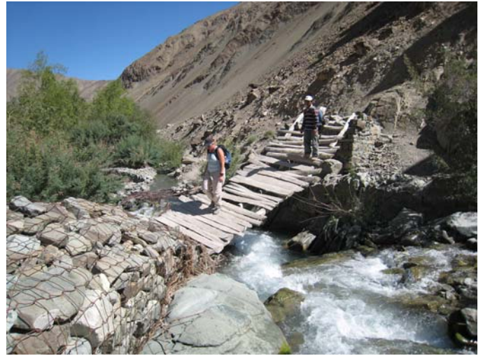
Bridge over the Jingchan
