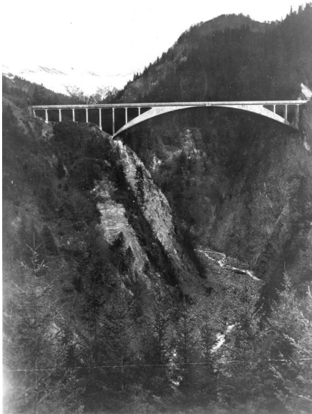
Fig. 1. Salginatobel Bridge, Schiers, Switzerland (photo reprinted with permission from Madame Marie-Claire Blumer-Maillart)
